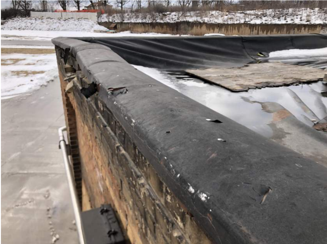
REMOVE EXISTING PARAPET CAP
