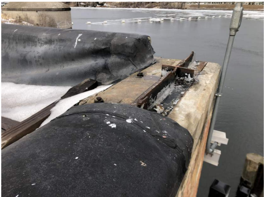
REMOVE EXISTING PARAPET CAP
